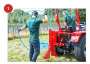
Set the pipe layer to the desired height, then feed the pipe slowly into the pipe layer.
